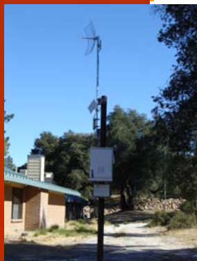
Microwave antenna installation at Casey Hall, providing Wi-Fi.
